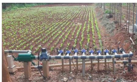
IoT pump controller
