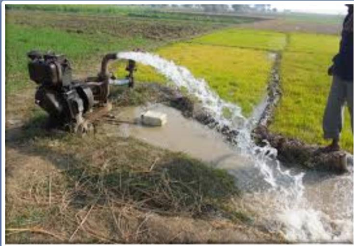
Electric Pump sets
