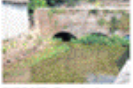
SUPPORT: Groundwater is pumped into the flow or 'thick' in Dorset to maintain healthy flow.
