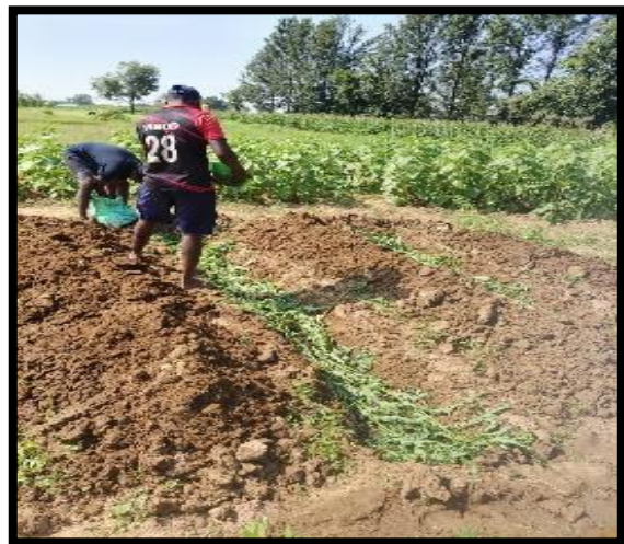
Filling the trenches
