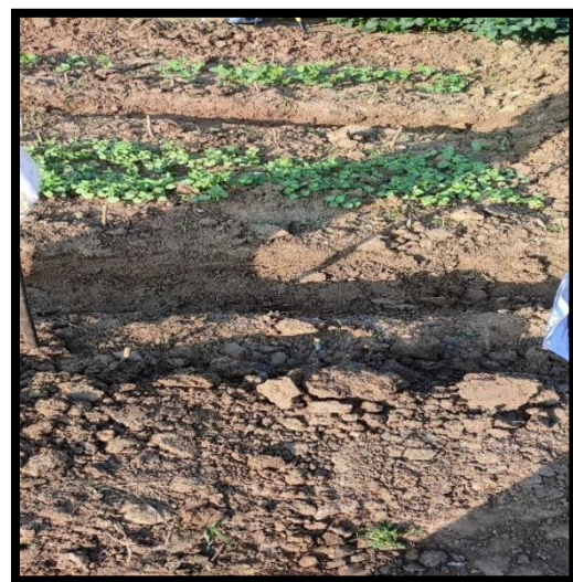
Trench for water harvesting & a filled trench
