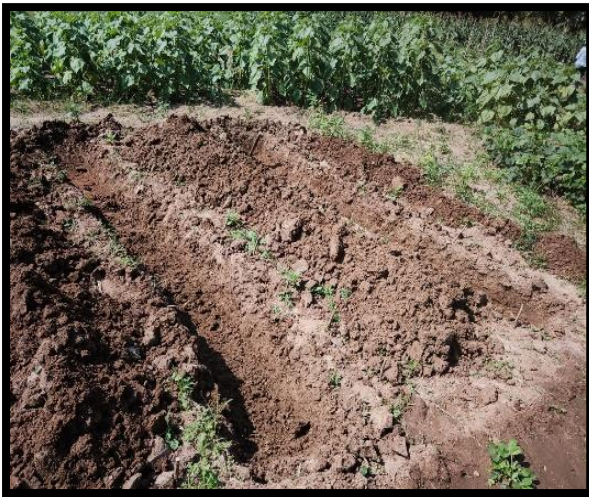
Digging of trenches
